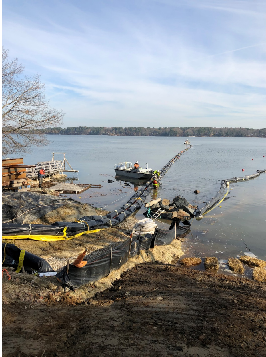
Mackworth Env preparing second turbidity barrier for transport to the eastern shore for installation. November 26, 2019 at 1155h.
